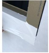
Cut tape at face of jamb legs, and fold up past interior corner and across outside face of jamb
