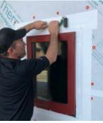
Roll the tape, to ensure a good air & water seal.
