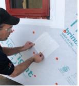
Insert repair block into opening, ensure snug fit.
