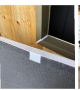
**TAPE FLAP** Apply small strips of flashing tape to the flap to adhere to the Neopor insulation.
