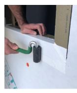
Adhere the tape from sill down and over the ThermalBuck and onto WRB.
