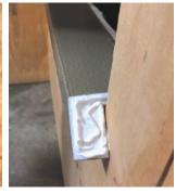
SEAL ENDS Add sealant to mitered ends.
